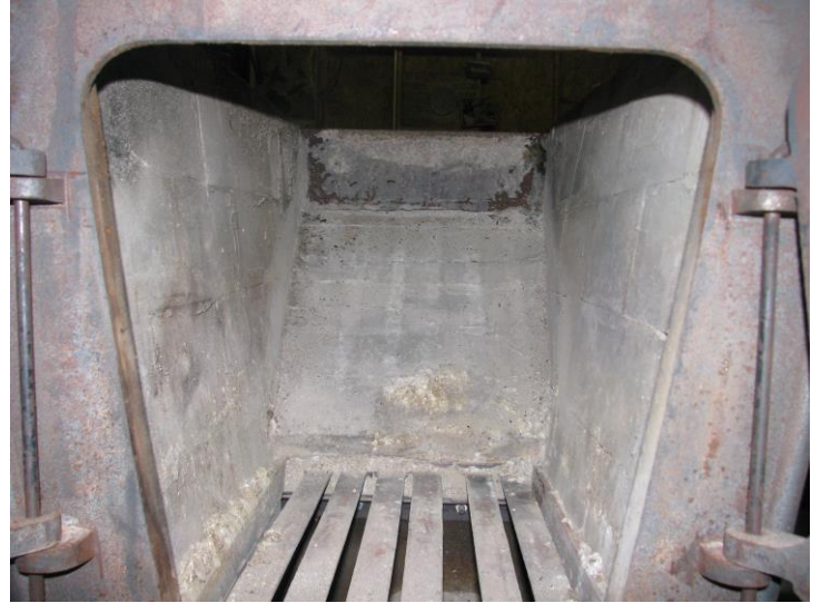
Insulation board laid out in the arch
